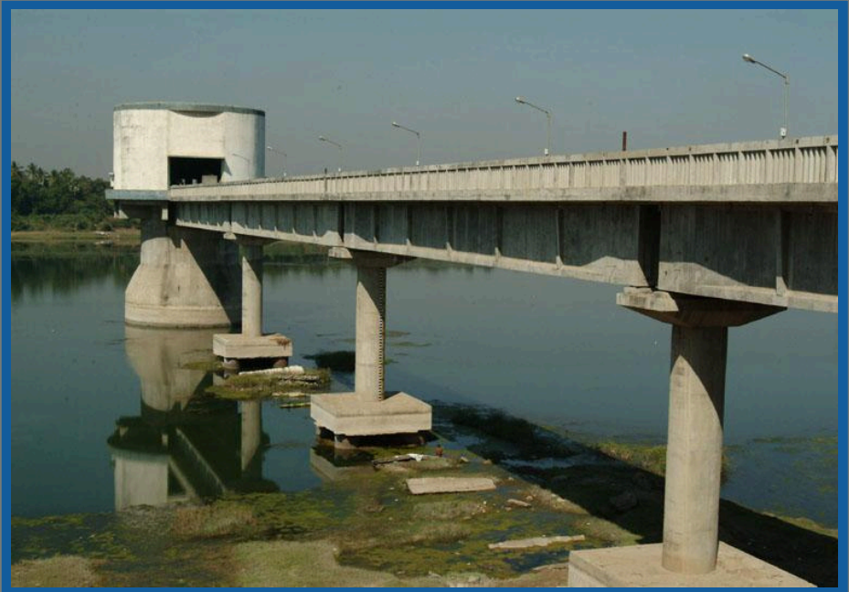
Approch Bridge with Intake Well
